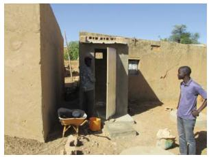
Project Manager Serigne Madjou (r) inspects the work on the biodigester project for one household in Guédé Chantier. One of the workers (l) is making sure that the door to the Turkish toilet fits and locks. On the ground can be seed the concrete components of the biodigester system. When the system is completed it will provide biogas that can be sued to cook the food for a household, eliminating the need for burning wood.
