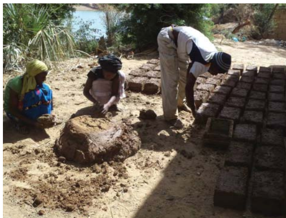
Members of the Eco-Sentinelles of Guédé Chantier, Senegal form mudbricks that were set out to dry and then used to add a new classroom to one of the community's elementary schools.
